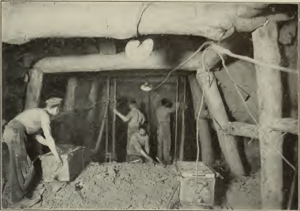
FIG. 20. ROTARY MINE DRILL ELECTRIC-DRIVEN THROUGH FLEXIBLE SHAFT.
